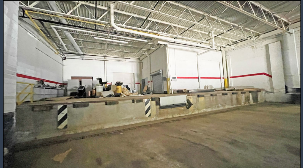
INTERNAL LOADING AREA
