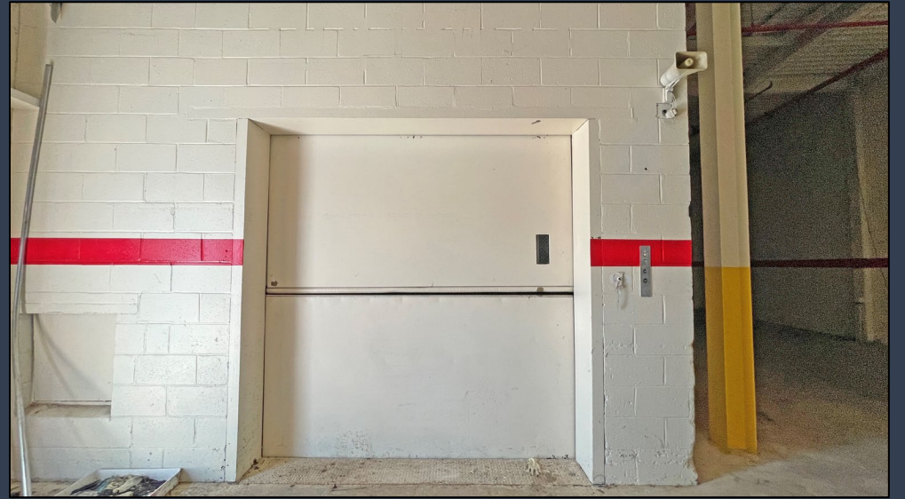
FREIGHT ELEVATOR (needs 200 amp electrical hook up)
