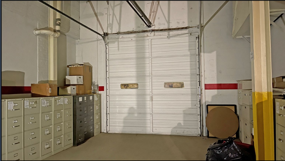
INTERNAL OVERHEAD DOOR
